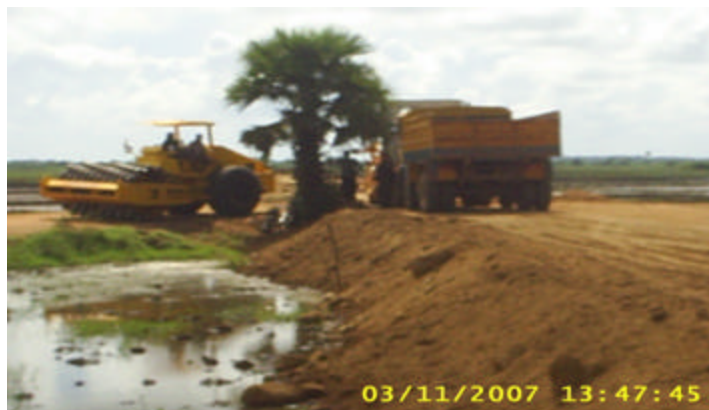
Road being built across the paddy fields
